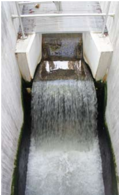
Treated wastewater from a treatment plant provides high-quality water for paddlefish culture.
